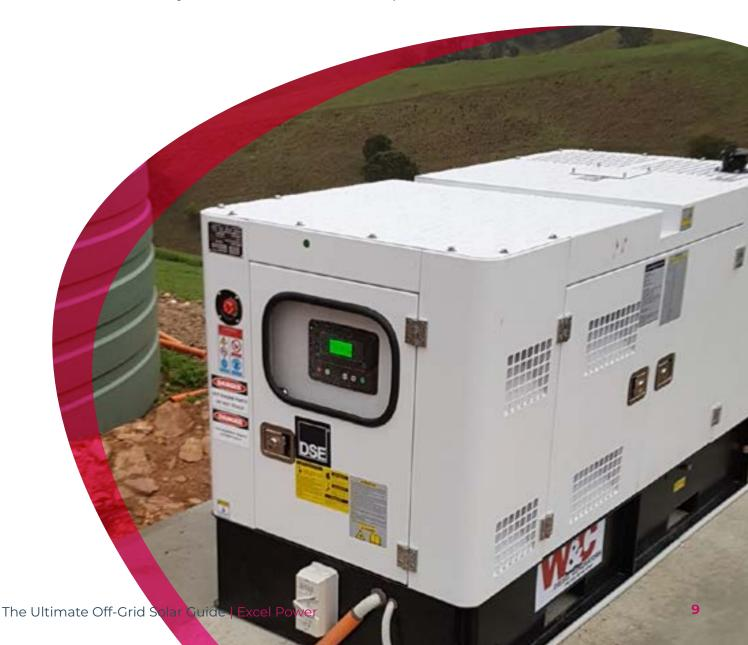
**Economic considerations in cloudy regions** - In areas with frequent cloudy weather, an excessively large solar and battery system is not cost-effective. Combining solar, battery, and a backup generator is a more cost effective and professional solution.
