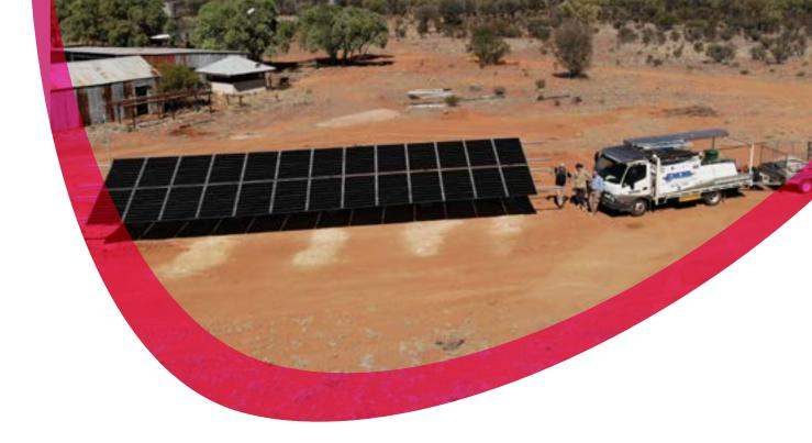
**Sunlight and panel placement** - Assess sunlight availability, considering shading from structures or trees and your area's climate. Our specialists will identify the best location, orientation, and tilt for solar panels to optimise efficiency. If your roof is small, consider a free-standing array, though it may increase costs.
